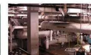
Draining water from the basement
